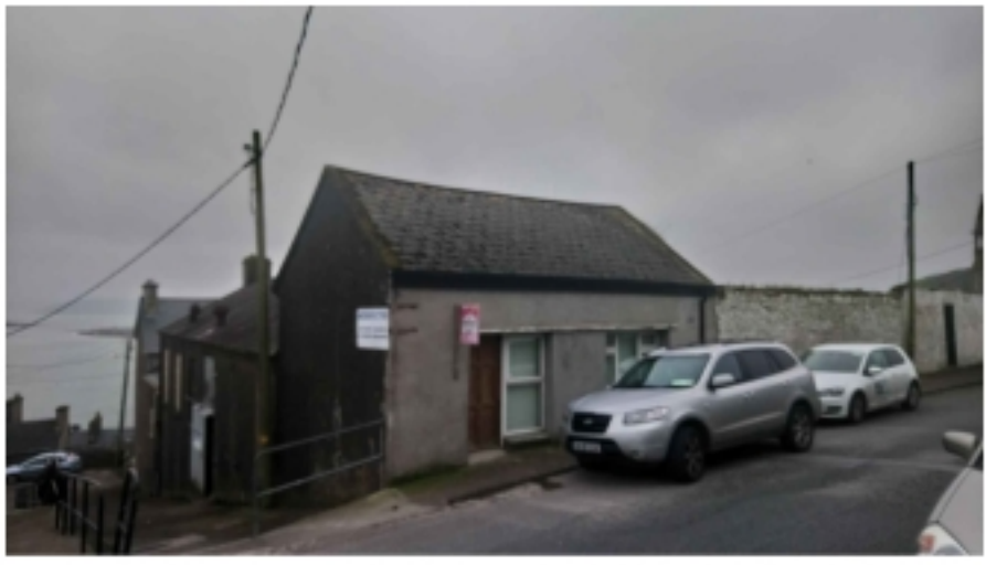
THE EXISTING BUILDING
